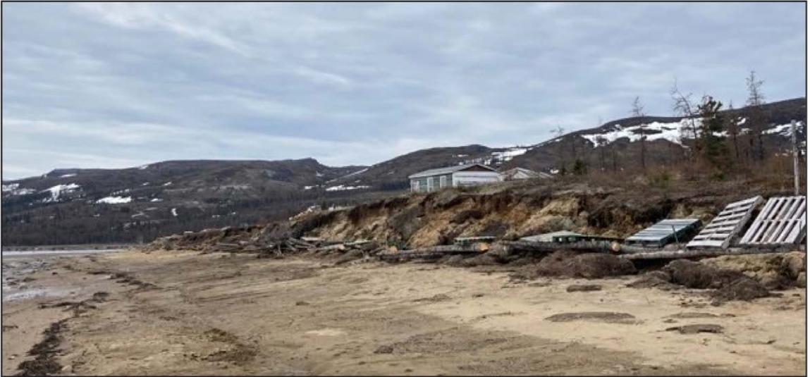
A view of the beach and bluff with pallets and logs positioned to absorb wave impacts and reduce erosion near the Webb family's homes on Webb Bay.
